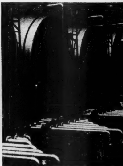
TANK STORAGE —Battery of Nordstrom valves control flow of gasoline, butane, and propane from storage to loading racks.
